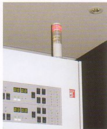
Built-in Computer System
